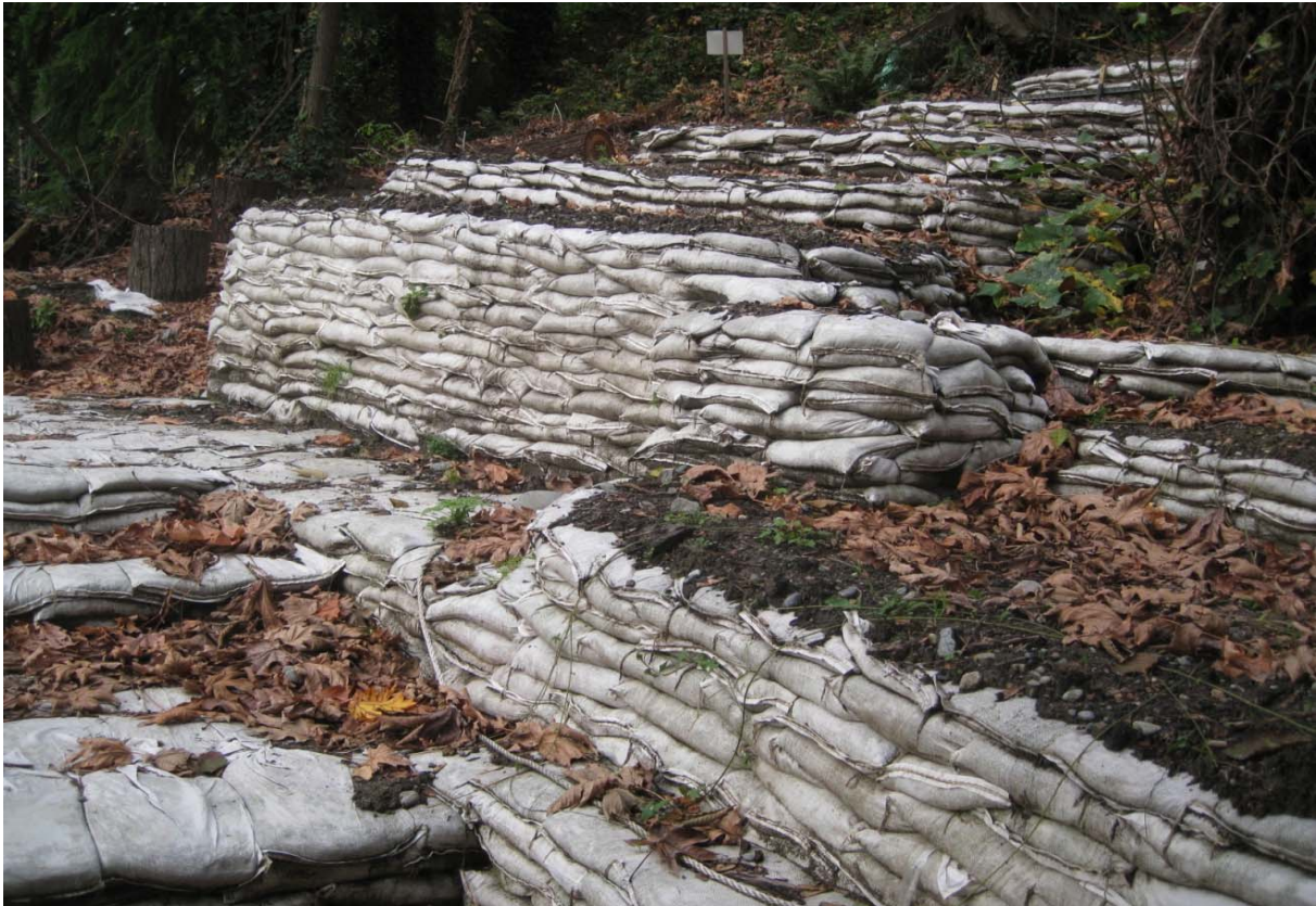
Photo #5: View of tiered sandbag walls on the project site (Nov 11 2016).
