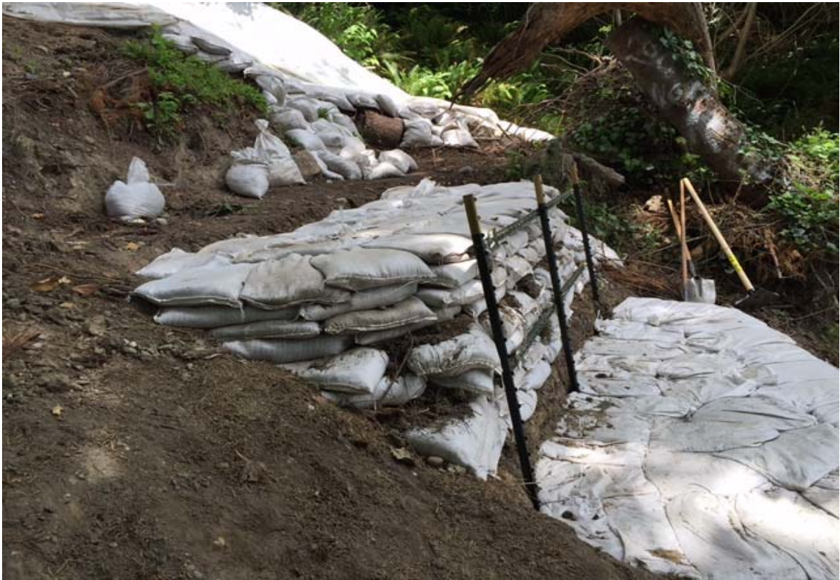
Photo #19: Continued construction of upper sandbag walls (May 17 2016).
