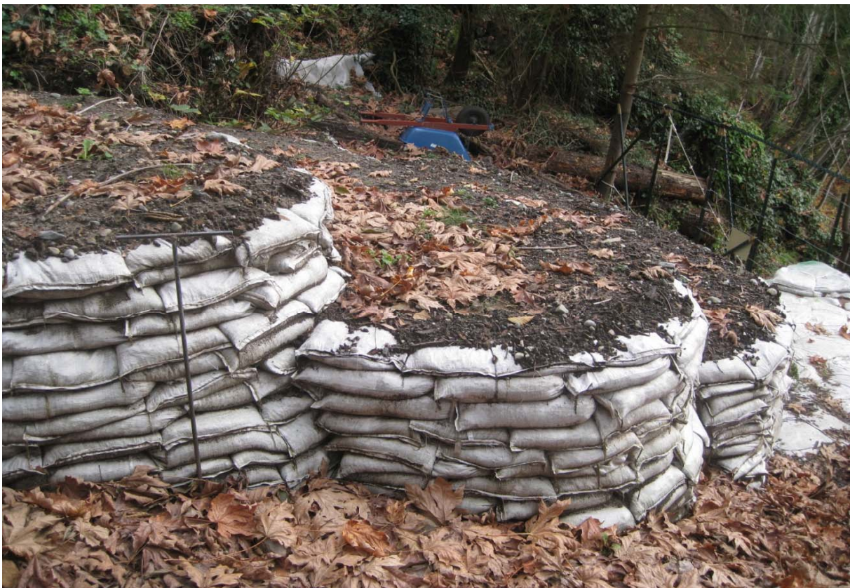
Photo #8: Downward and eastward view of the upper sandbag walls (Nov 11 2016).
