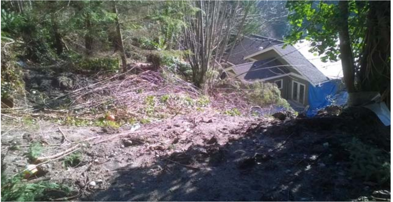
Photo #15: Downslope view of slide area on site property (Feb 2 2016).
