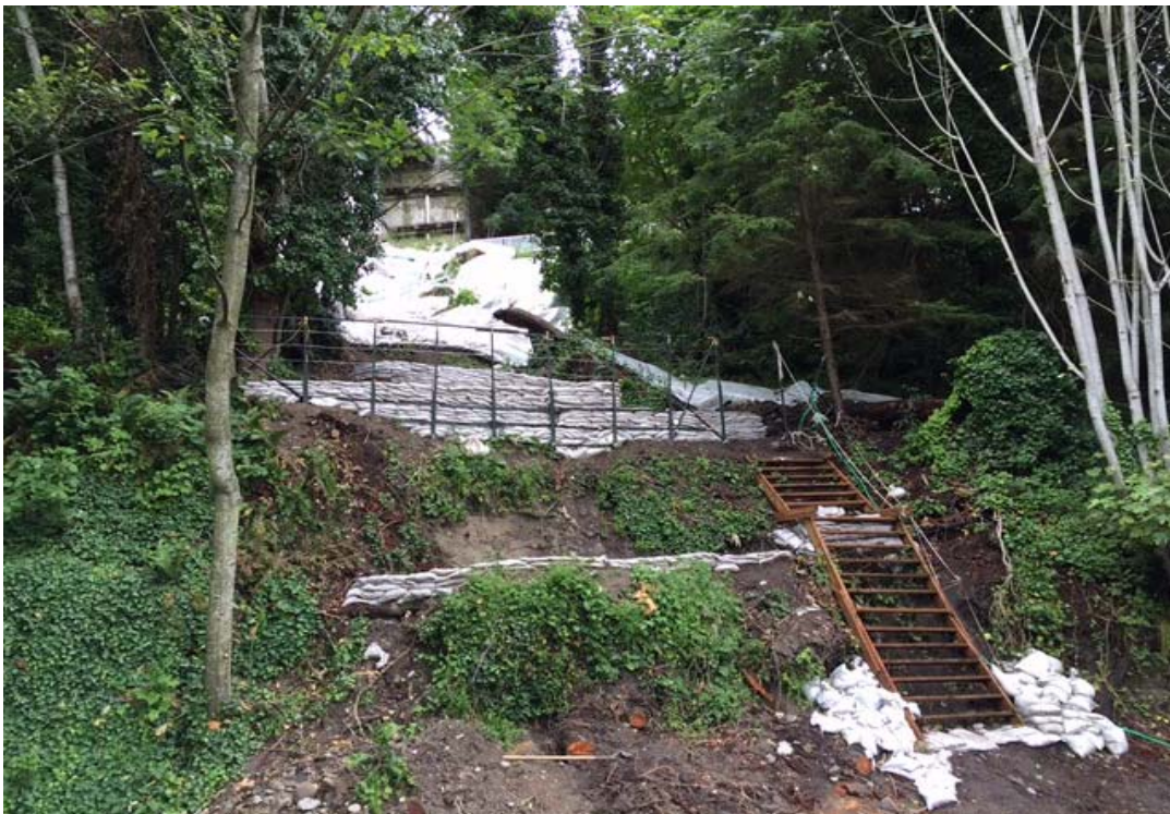
Photo #24: Completed lower sandbag walls (May 25 2016).
