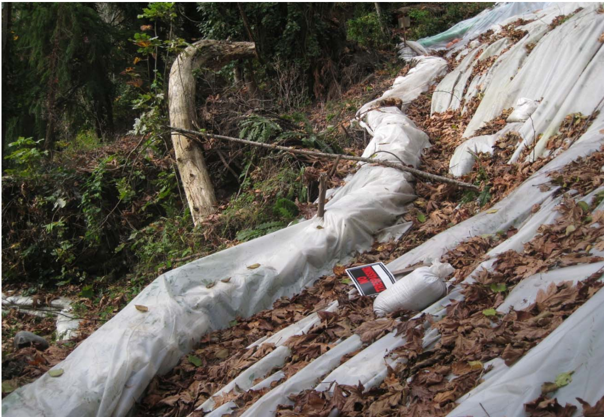
Photo #14: Westward view of sandbag berm and plastic sheeting (Nov 11 2016).
