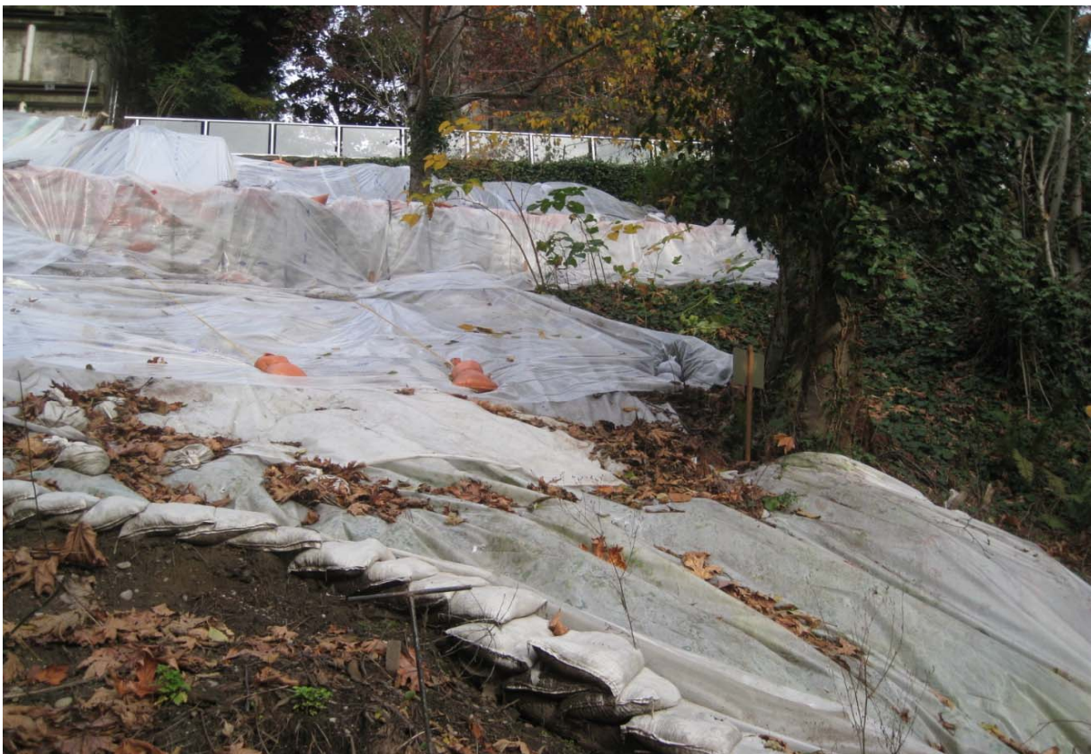
Photo #12: Sandbag berm and plastic sheeting on northern margin of site and adjacent properties (Nov 11 2016).
