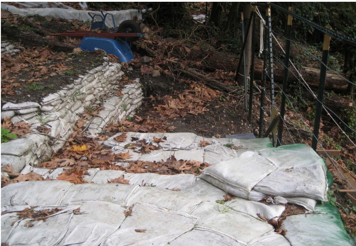
Photo #6: Eastward view of the lower sandbag walls (Nov 11 2016).
