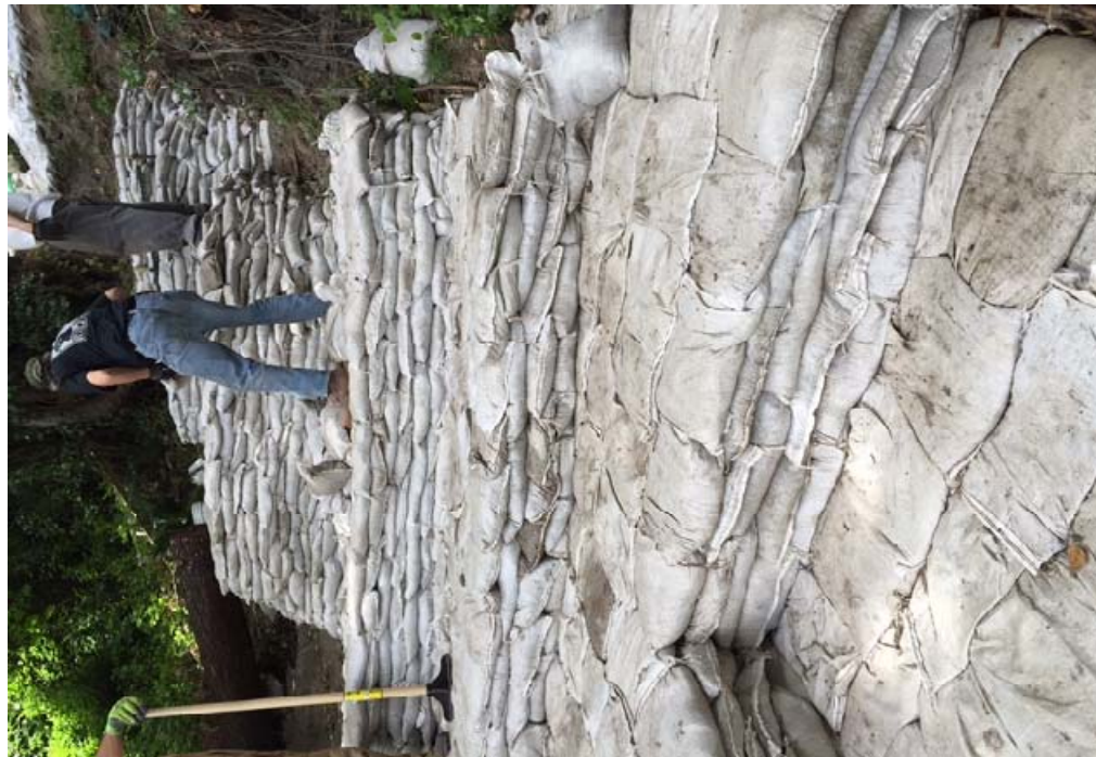
Photo #21: Construction of upper sandbag walls (Jun 2 2016).
