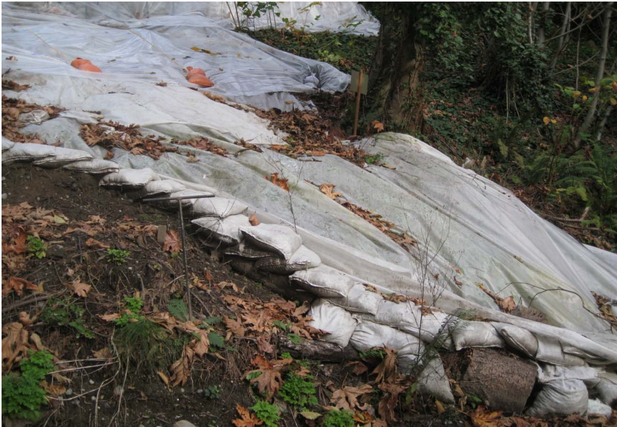
Photo #11: Eastward view of plastic sheeting and sandbags on adjacent north property (Nov 11 2016).
