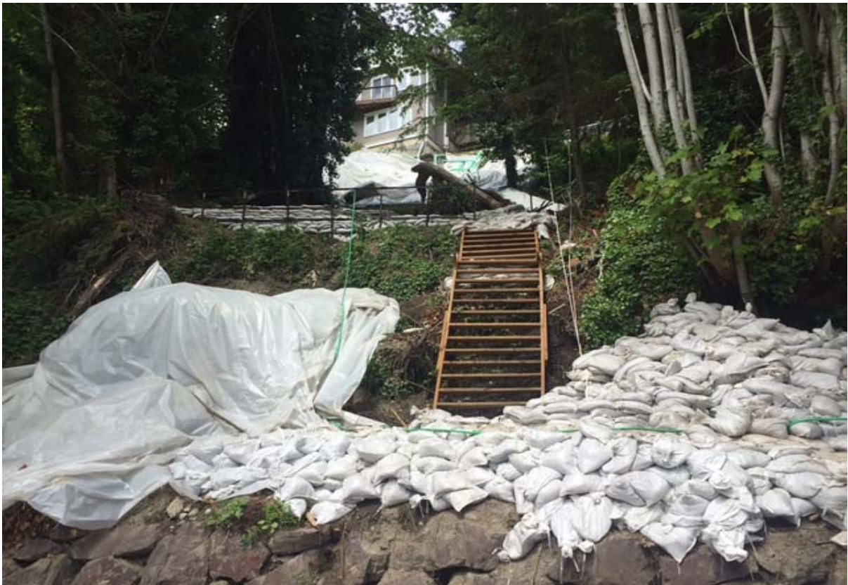
Photo #20: Construction of lower sandbag walls (May 25 2016).
