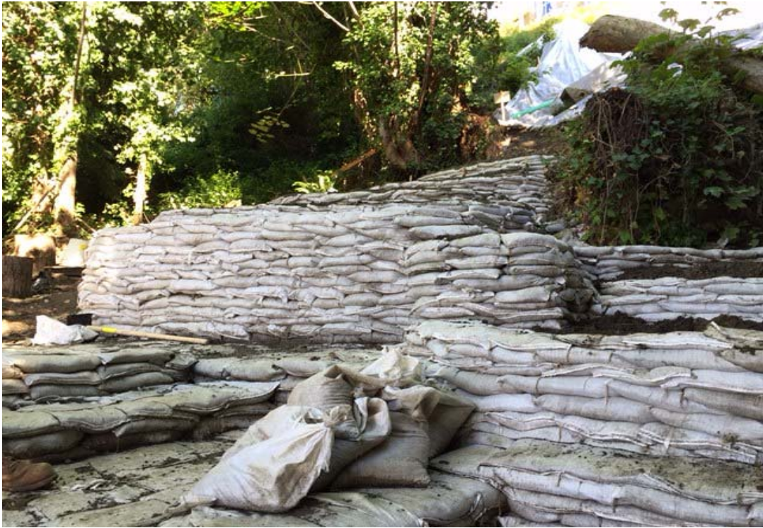
Photo #23: Completed upper sandbag walls (Jun 22 2016).
