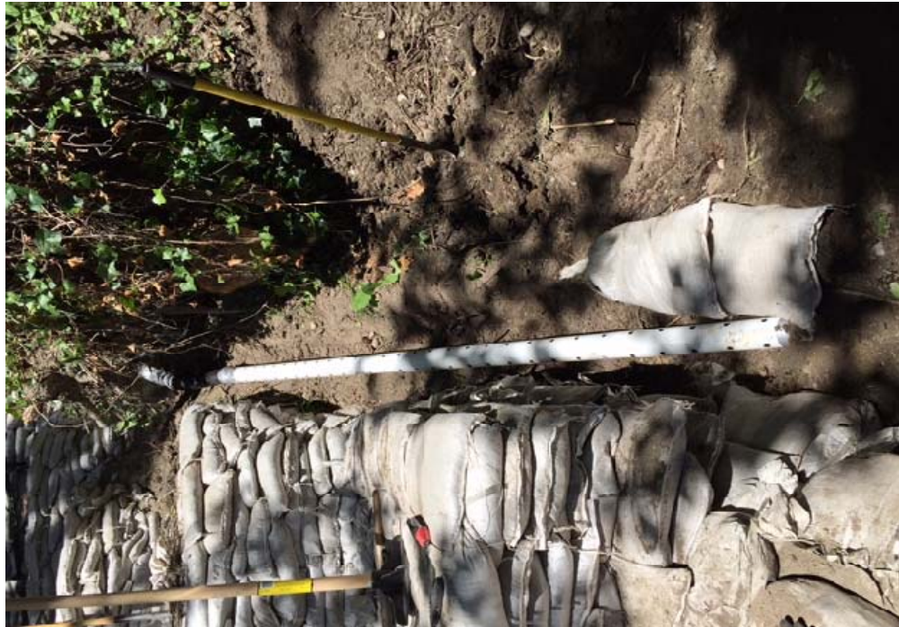
Photo #22: Subsurface drainage next to upper sandbag walls (Jun 6 2016).
